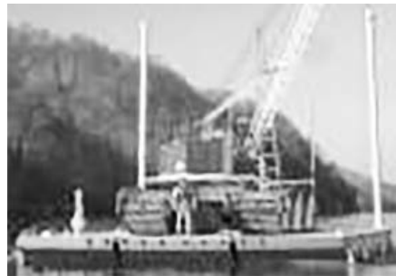
32' x 40' x 4' Sectional Spud Barge and Crane.
