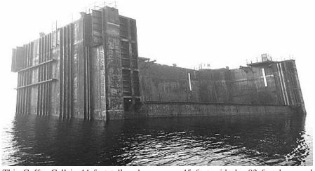
This Coffer Cell is 44 feet tall and measures 45 feet wide by 93 feet long and weighs 640 Tons. The Coffer Cell could serve as a portable drydock, potential breakwater, and more. The Coffer Cell was used on the SR 520 Floating Bridge, to provide a work platform. We can provide as-built drawings. Price on request. It is currently located off the shores of Bellingham, Washington.
