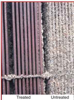
Before / After An example for the impact on a professionally used Boxcooler, with and without the treatment by our ultrasonic solutions.
