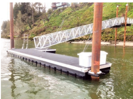
RESIDENTIAL DOCK WITH FIBERGLASS GRATING DECK
