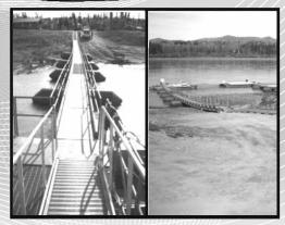
Portable military surplus Bailey Bridge. Used on the Yukon River in Eagle AK. 200' of ramp, two floating platforms approx. 12' x 24', Ramp sections are 4" wide by 11' or 22' long, approx. 100' of galvanized hand rail. 4' x 16' steel pontoons.
